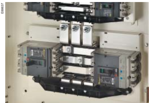
NS/NB branch breaker extension 2 Ways
